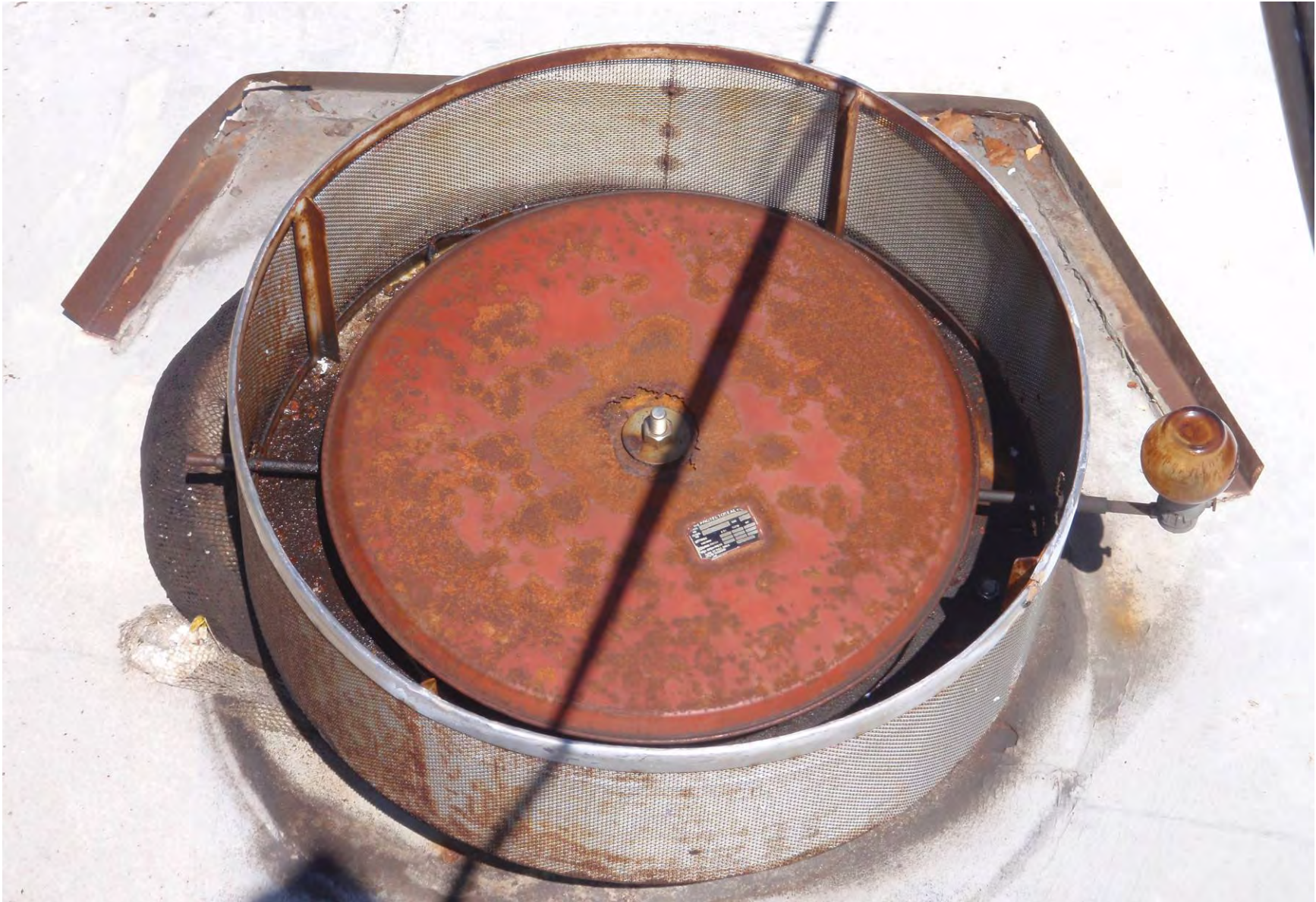
The 20" Emergency Hatch (PSV-294B)
