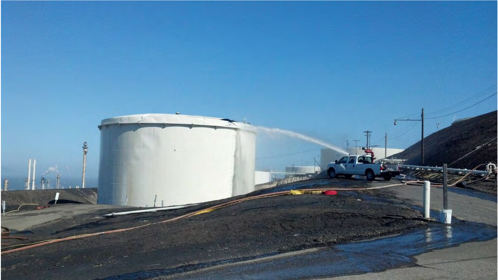
Tank 294 during the initial emergency response.
