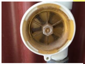
Rotary Flow Switch
